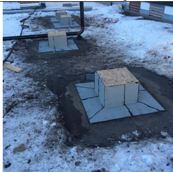
4.12- New roof penetrations on existing roof.
