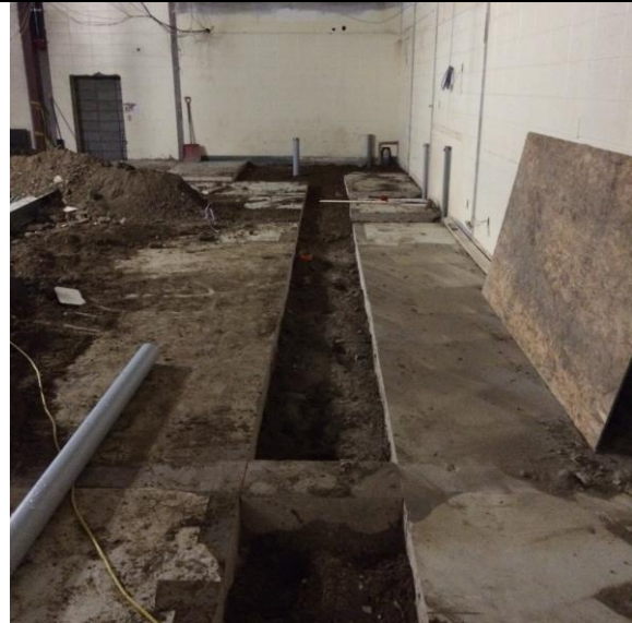
4.2- Food Studies u/s Plumbing being backfilled
