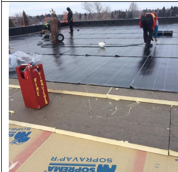
4.11- Gym Roofing progressing.
