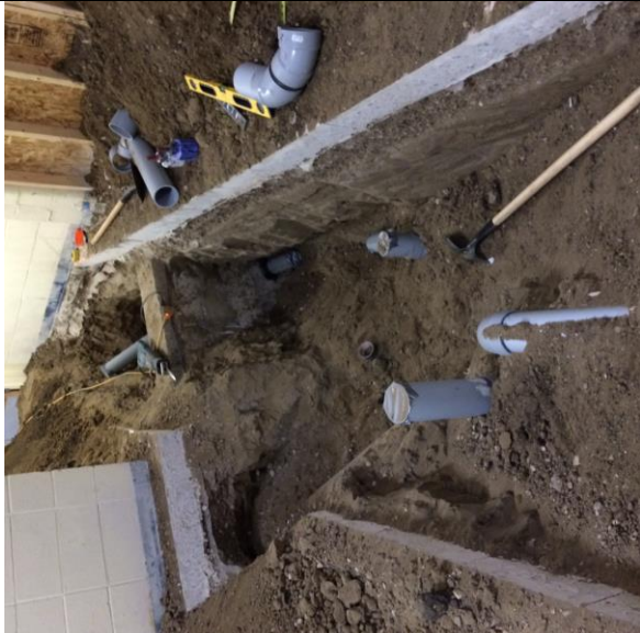
4.7- Commercial Kitchen u/s plumbing in progress.
