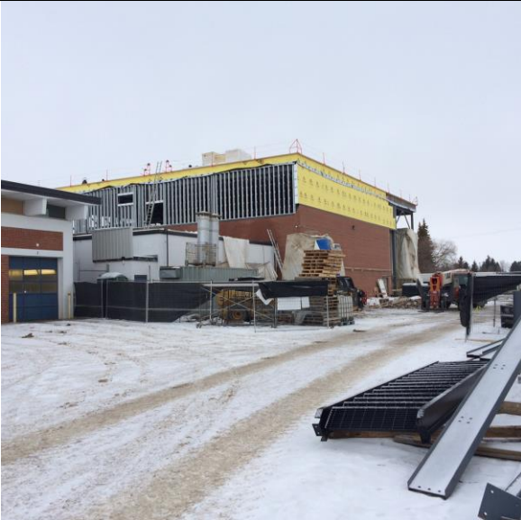
4.8- Gym steel metal stud walls.
