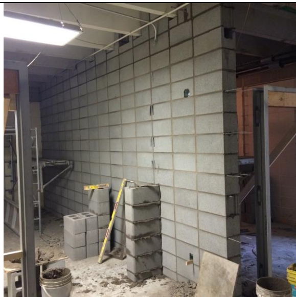
4.4- Block partition in Change Rooms
