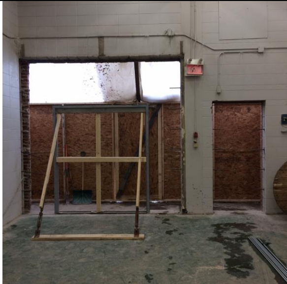
4.5- Electrical Room wall infill
