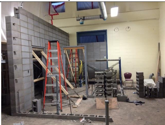
6.4- Concrete Block walls in Commercial Kitchen.
