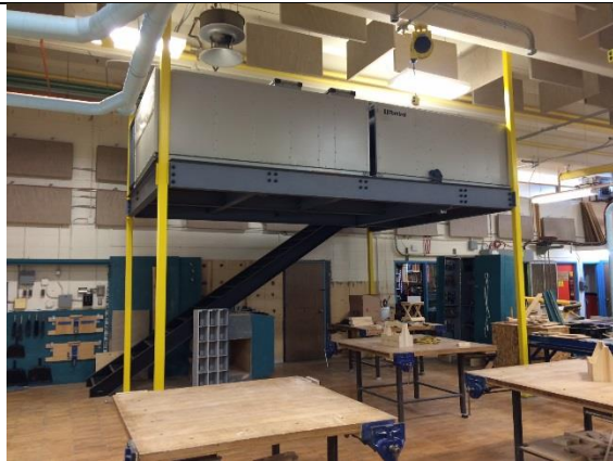
6.2- Shop Mechanical Platform columns painted.
