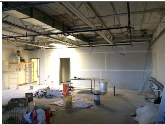
6.3- Drywall Taping in Science rooms.
